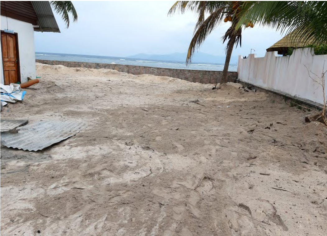
Site after construction of drain
