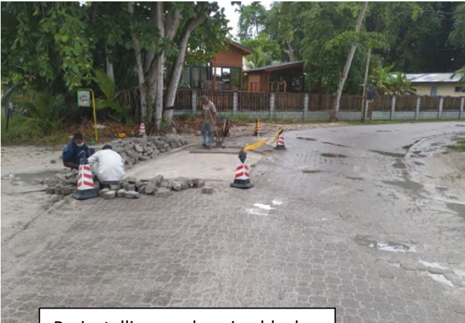
Re-installing road paving blocks along culvert.
