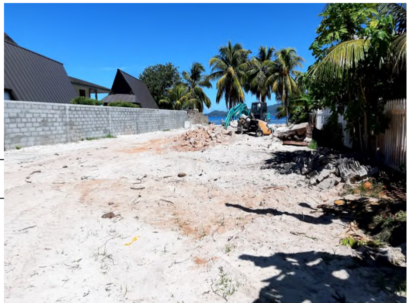
Drain along SPF plot -after
