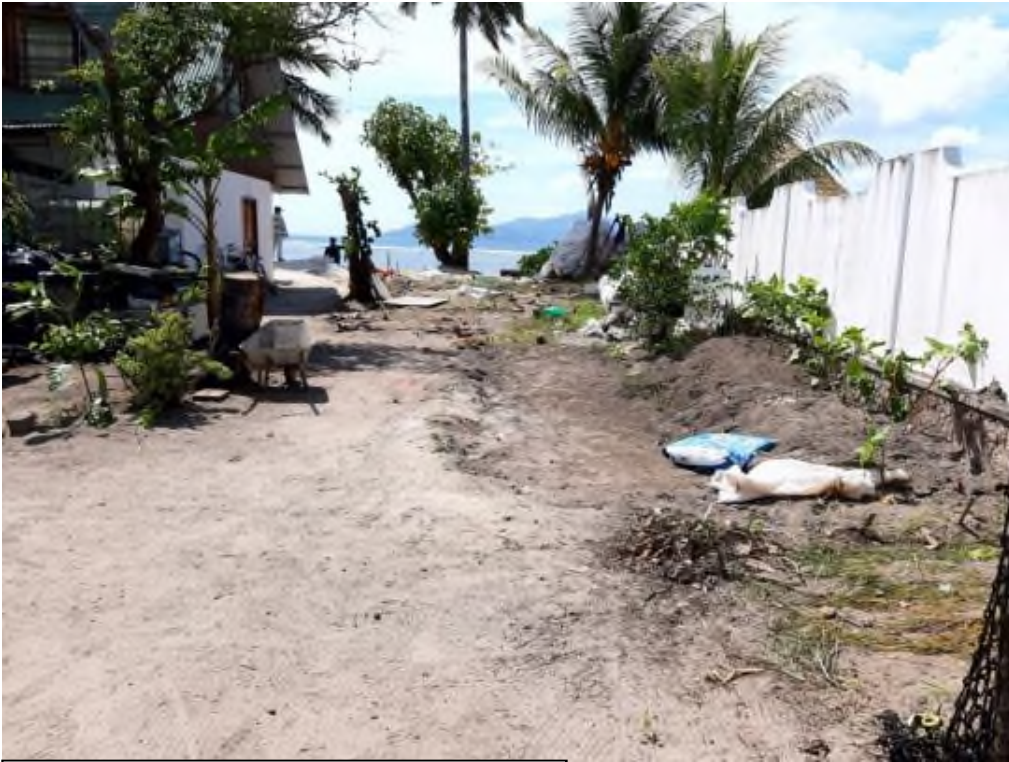
Site before construction of drain
