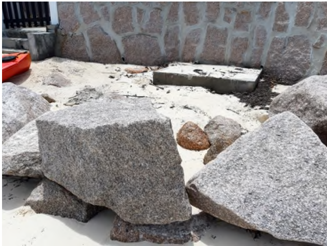
Drain outlet filled with sand at Outlet 3.
