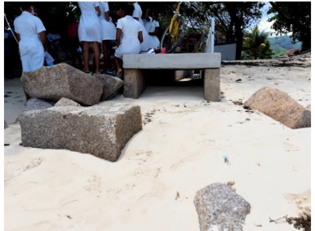
Drain outlet filled with sand at Outlet 4.
