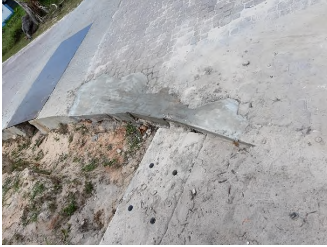
Road border completed at Outlet 3.
