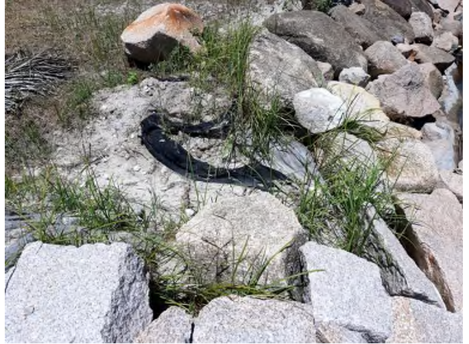
L'Union Estate excavated part of the rock armouring
