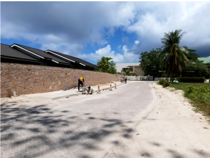
Finishing along road side.
