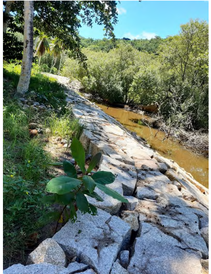
Rock revetment completed
