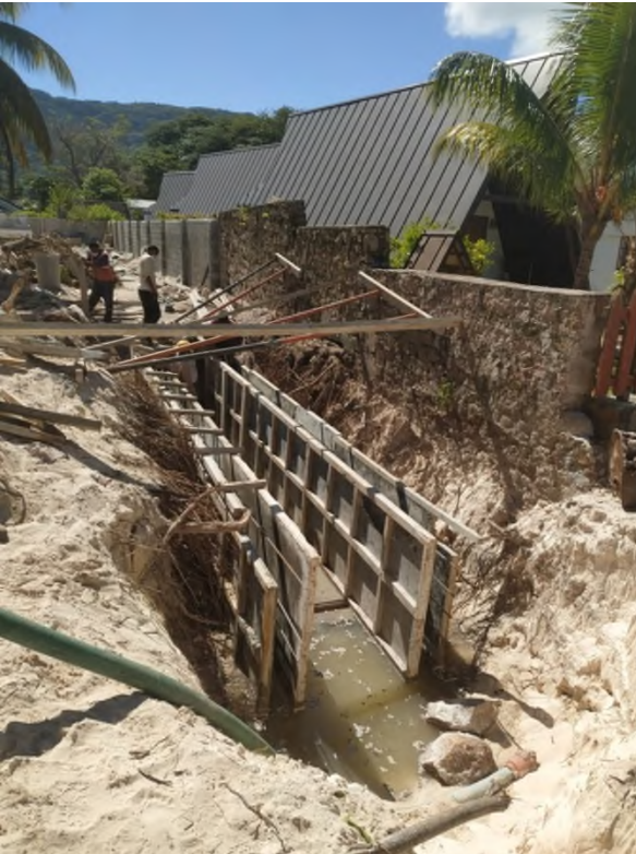
Construction of drain on SPF plot.
