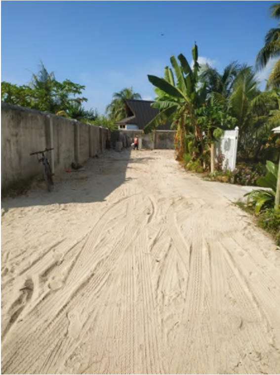
Drain from chainage 80 to 50 completed on 7 th March 2021.
