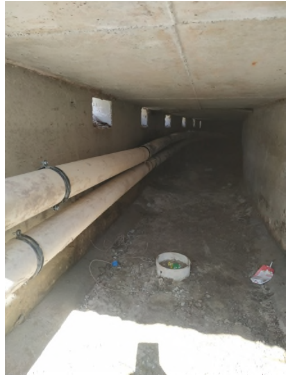
Installation of clamps for Cable and Wireless sleeves.
