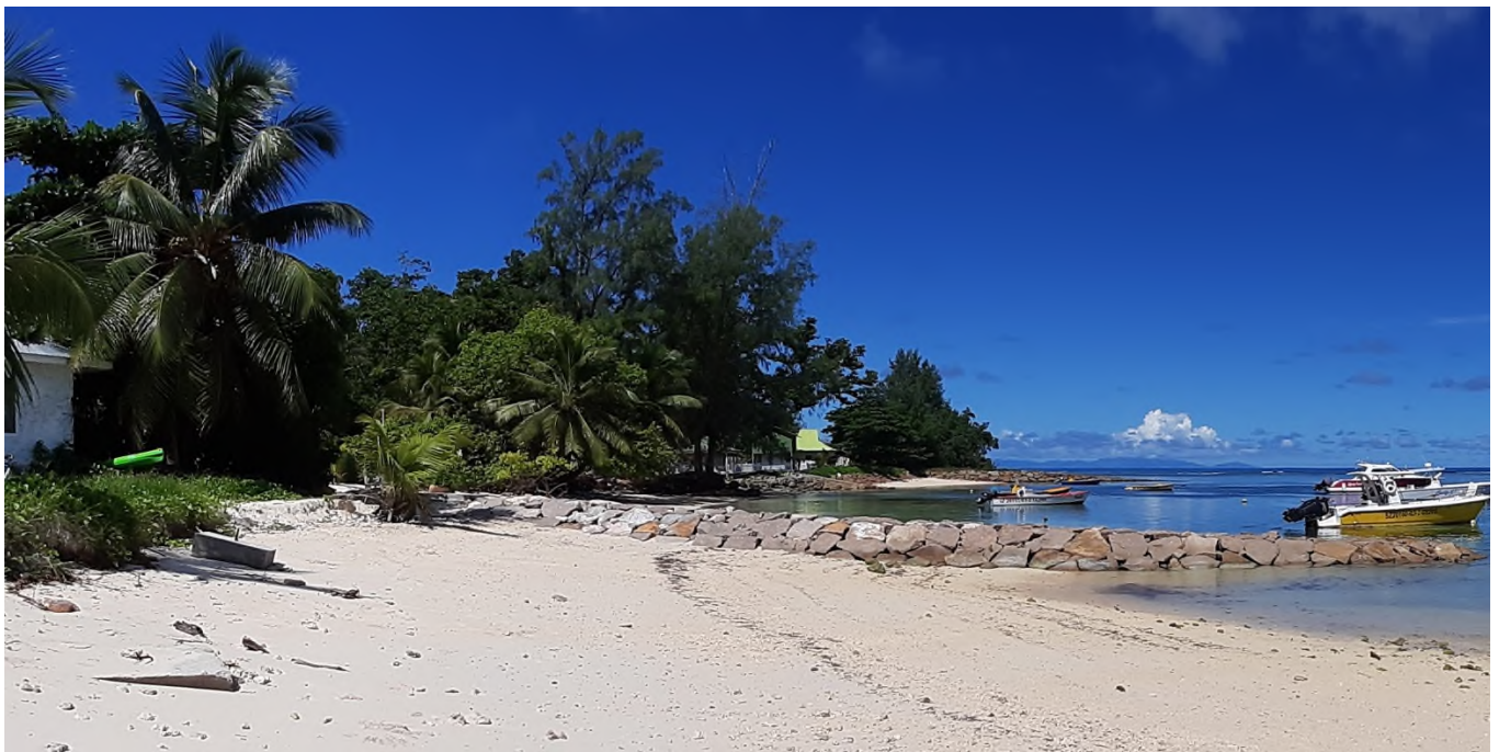
Newly constructed groyne.
