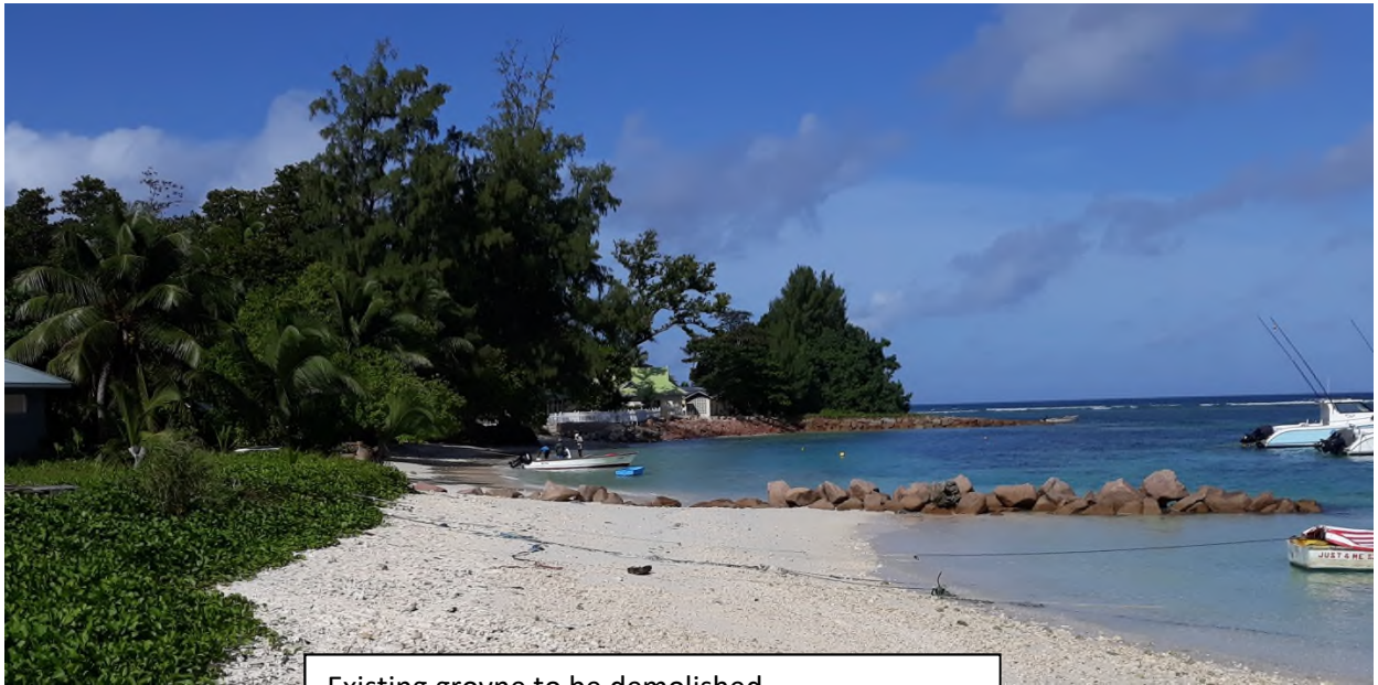
Existing groyne to be demolished.
