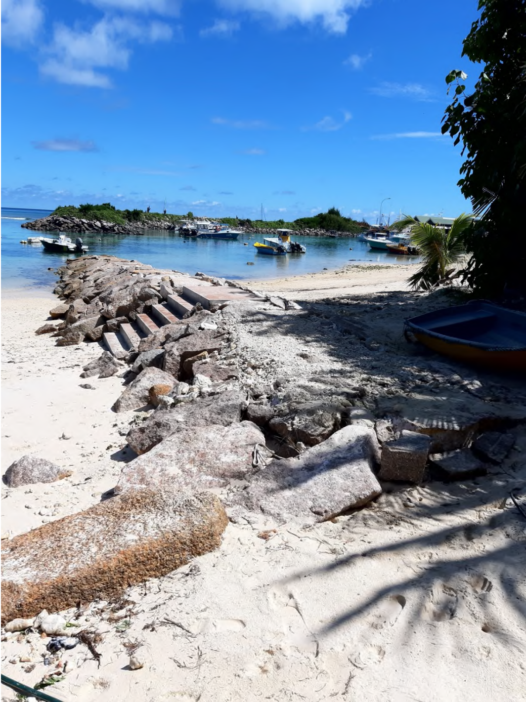
View of newly constructed groyne from Fishtrap restaurant.
