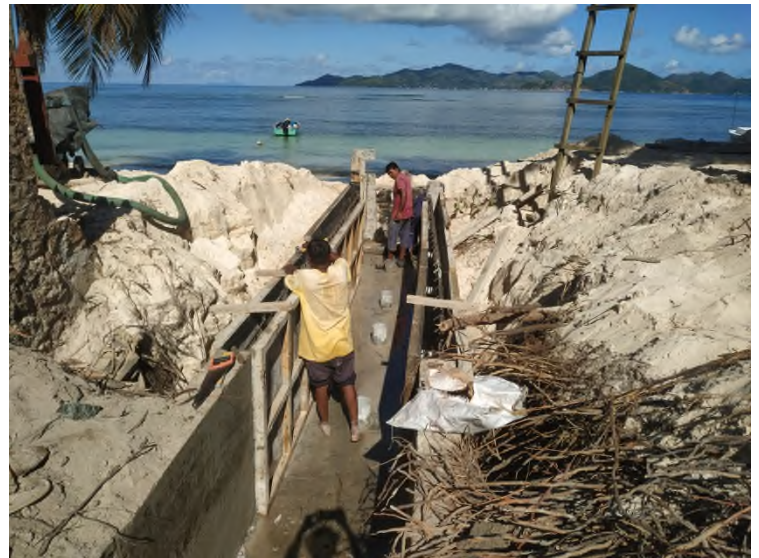
Extension of drain by 5metres to sea.
