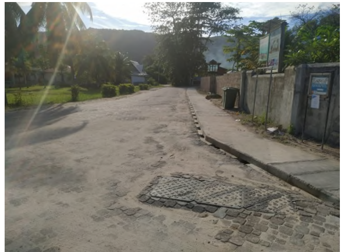
Works along road side completed on 4 th April 2021.
