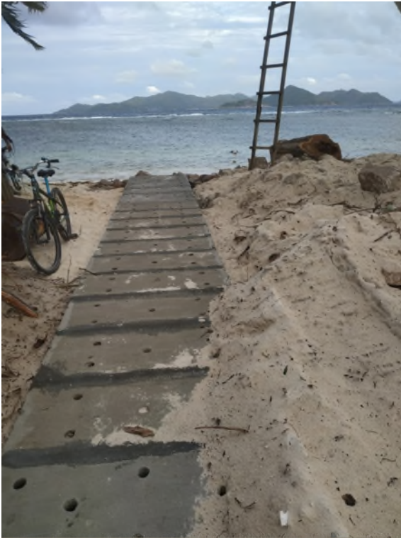
Cover slab over the last 10 metres of drain to sea.
